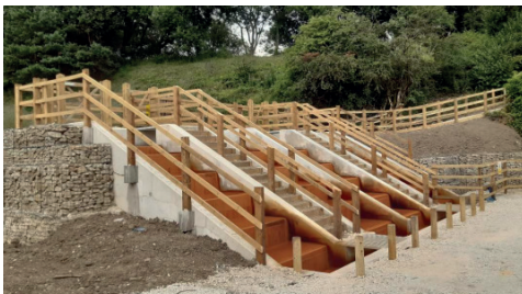
Figure 2 A recent cascade installation (2021) for a maximum flow rate of 80 L/s split into 4 cascades of 2 m individual width to aid in access of inspection and maintenance (Bullhouse, South Yorkshire)
