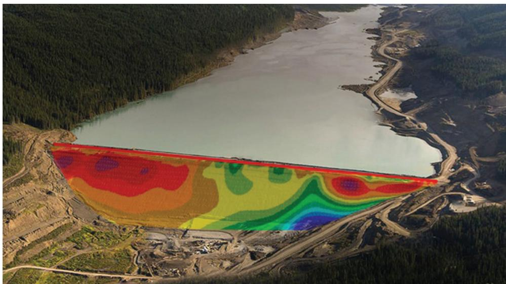
Figure 4 Permanent resistivity array installation to reveal weak zones in a dam wall (<https://www.lsi-lastem.com/products/G.Re.T.A./>)
