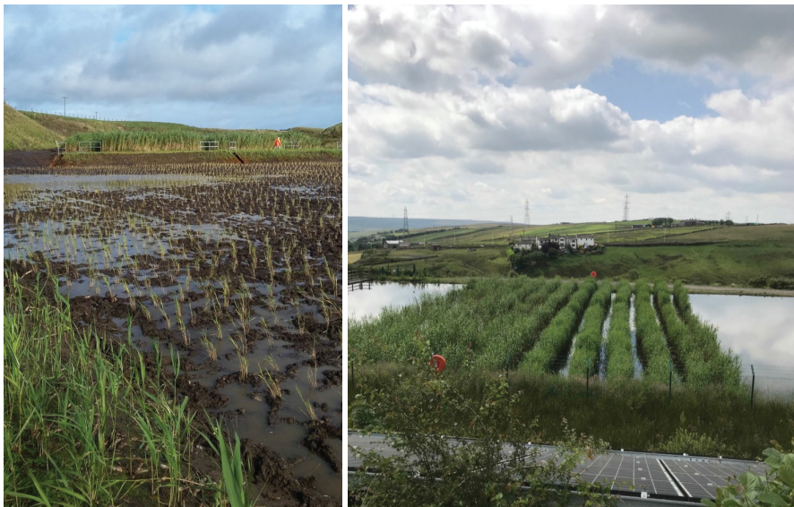
Figure 3 Individual planting of young plants at Pool Farm, Scotland (left), which failed to establish vs. acclimatised reeds replanted in rows at Deerplay, Lancashire (right)
