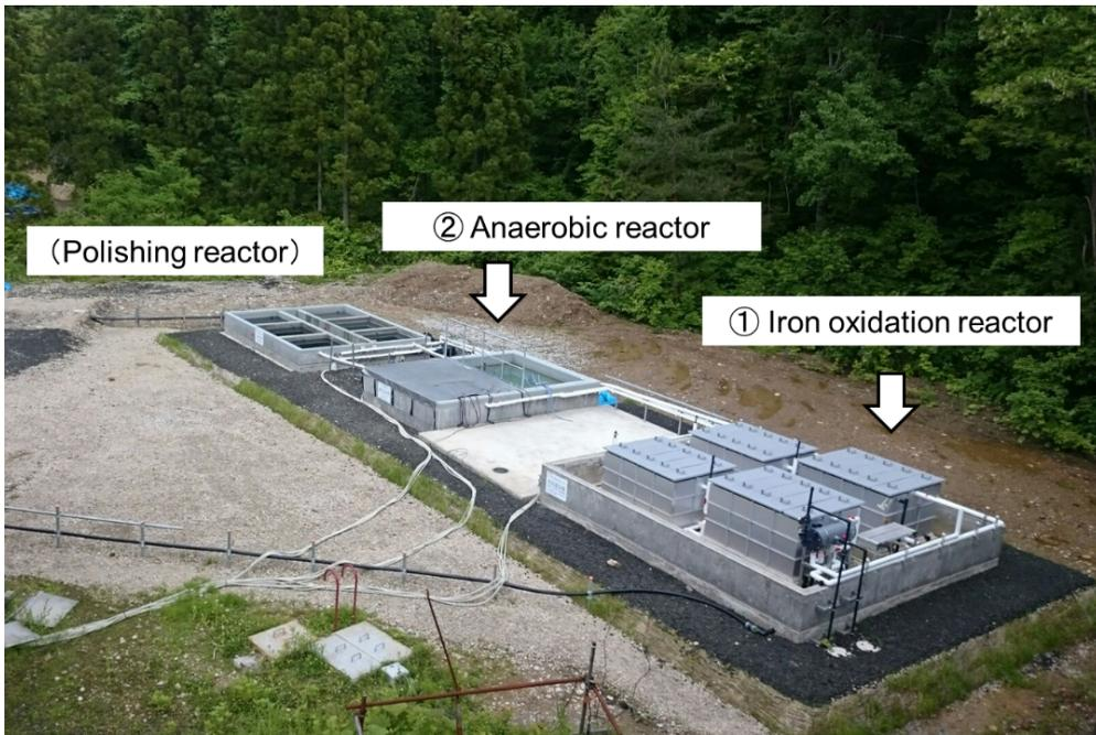
Figure 1 Pilot-scale demonstration test
