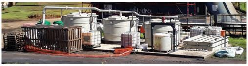
Figure 1 A view of the installed biological sulphate reduction pilot plant
