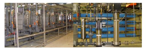
Figure 2 ED (left) and RO (right) in the GEAM plant (Toman 2009).
