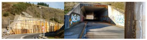
Figure 1 Anchor lines of a concrete retaining wall affected by corrosion (left) and ARD attack to precast concrete elements (right) along the newly-built AP-1 Highway. Guipuzkoa (Spain).
