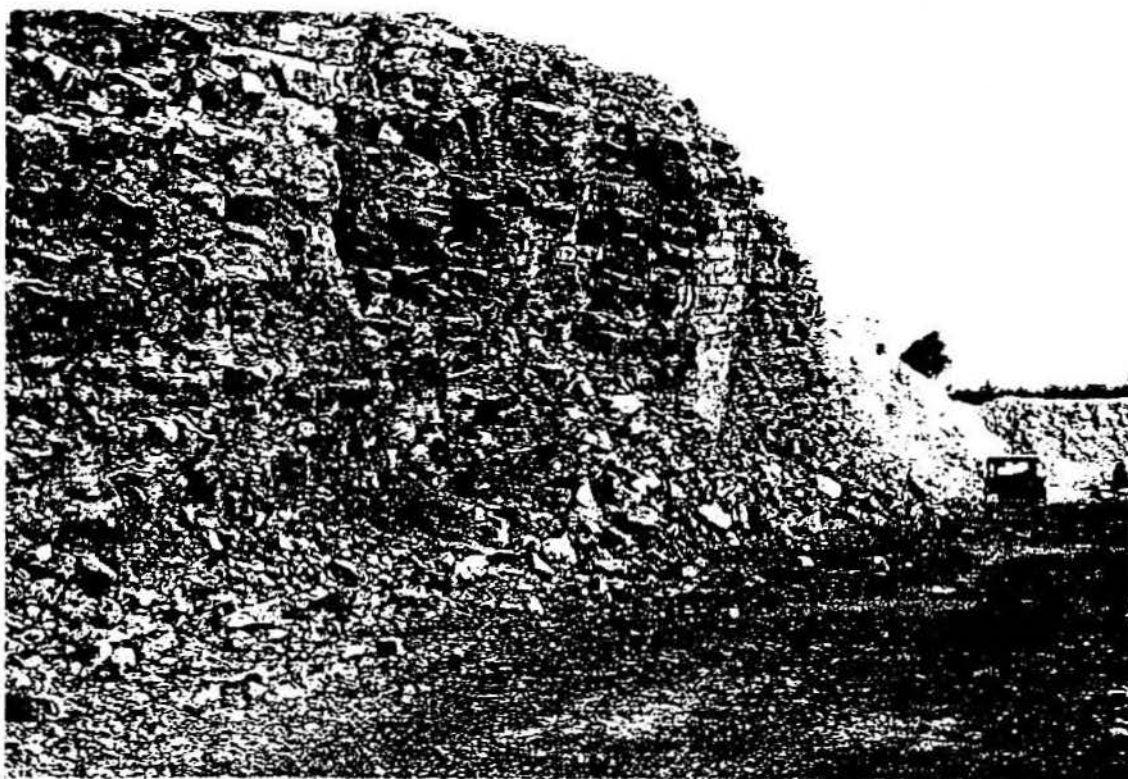
Photograph No 8 Bench B, N zone/W wall. Toppling failure
