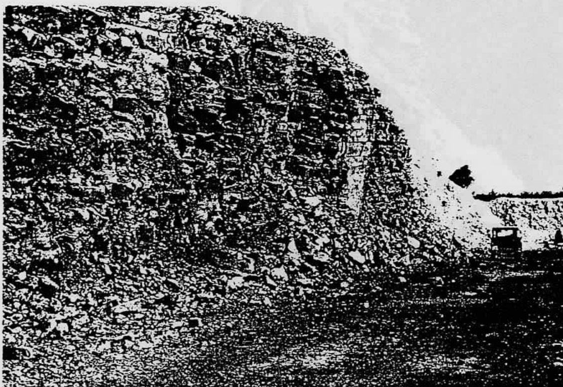
Photograph No 8 Bench B, N zone/W wall. Toppling failure
